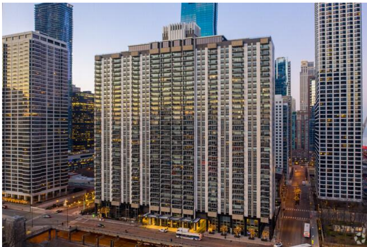
Figure 1. The Outer Drive East Condominium building is located at 400 E. Randolph Street in Chicago.
